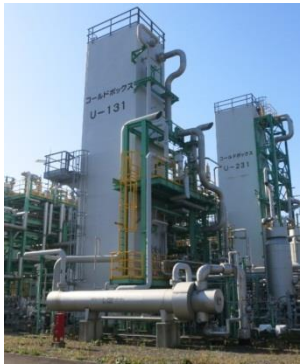
SSLNG Plant On Land
